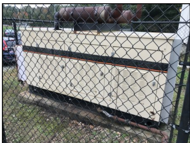
5 : Gas fired emergency generator
