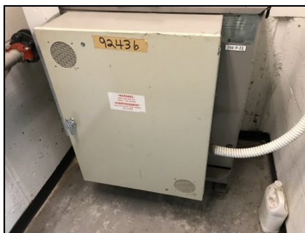
16 : Elevator hydraulic unit
