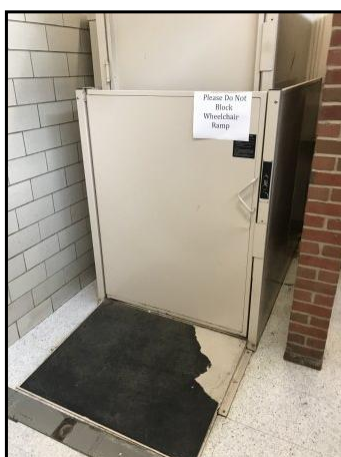
17 : Handicap elevator unit
