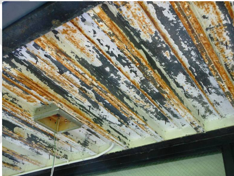
Exterior soffit with exposed metal deck and exposed abandoned wiring
