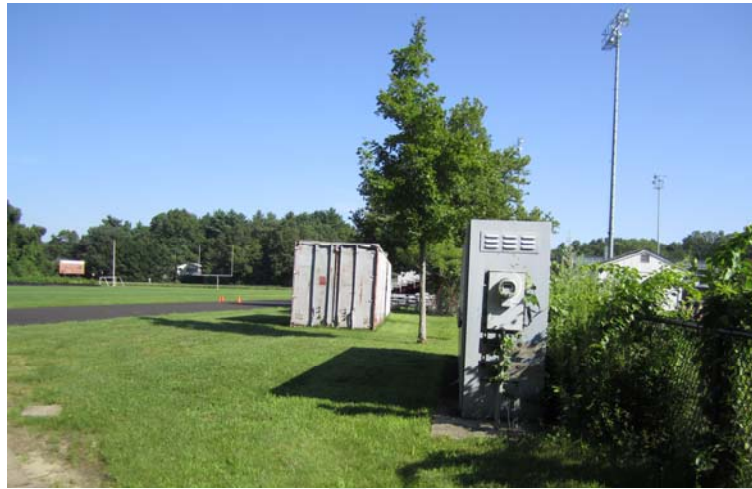
| Sport Lighting Power/Metering Enclosure
