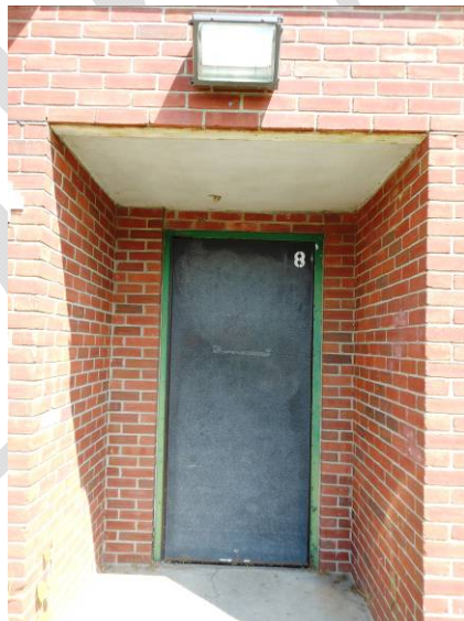
Gymnasium egress doors with lintel damage 1997 addition doors with rust damage above
