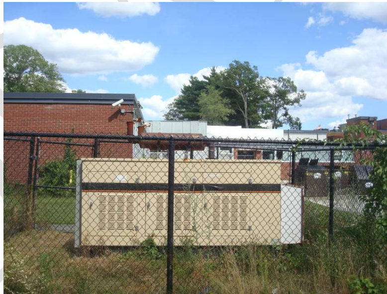
Natural gas engine-generator set
