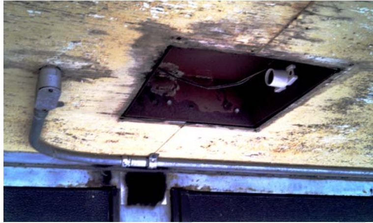
Exterior plywood soffit showing mold and abandoned light fixture
