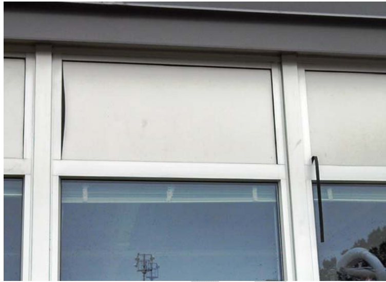
Missing and loose gasketing at storefront infill panels
