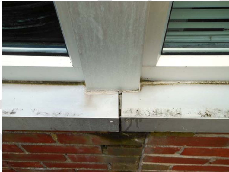
Storefront sill overlaps create water damage to wall below
