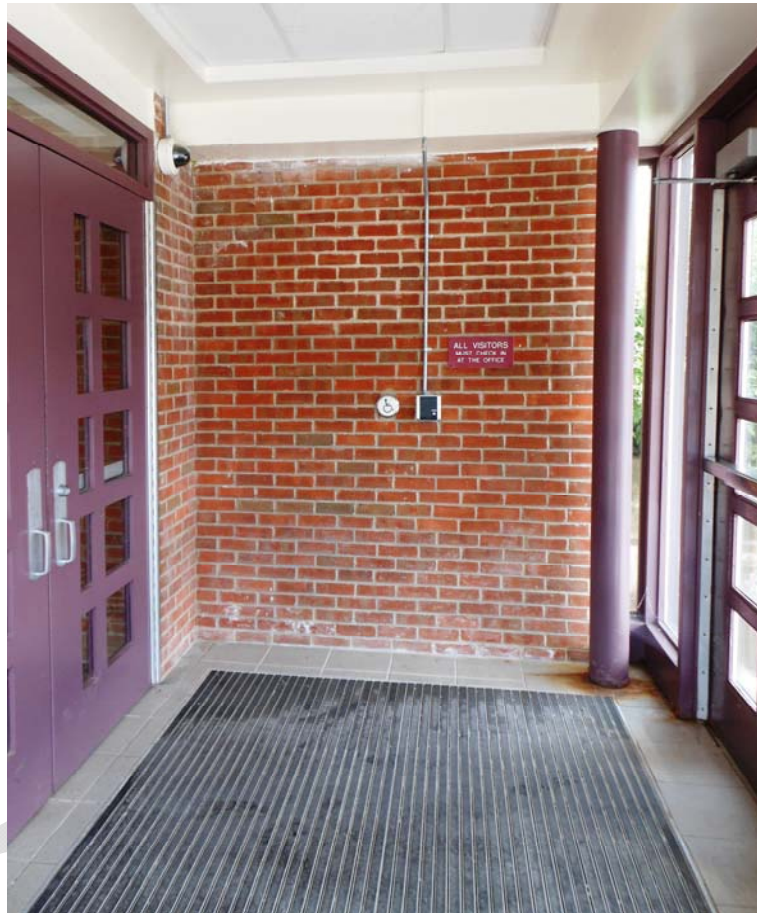
Automatic door opener and security at main entry doors
