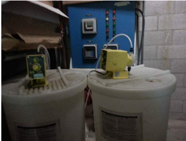
The pH is within a common storage room and has no ventilation or emergency shower.
