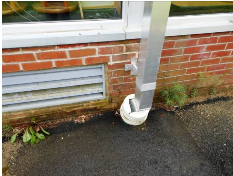
Scupper base at asphalt condition
