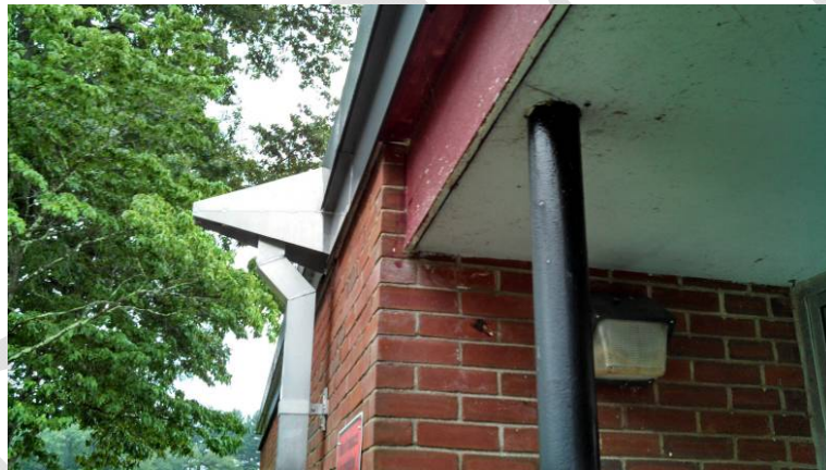
Exterior plywood soffit showing mold
