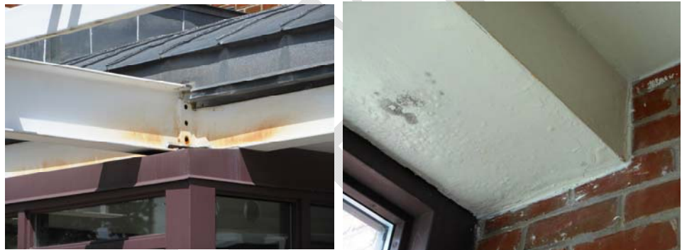
Mildew and bubbling at main entry soffit vestibule. Rust damage on exterior shows water infiltration.
