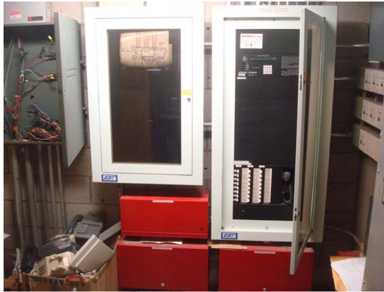
Fire Alarm Control Panel (FACP)
