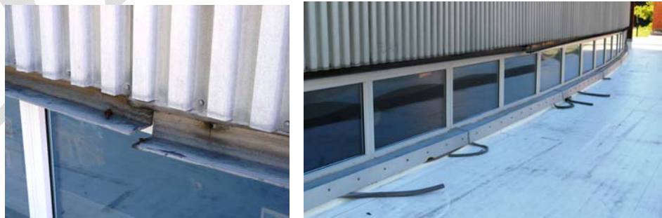
Damaged to exterior wall at Auditorium exterior - loose lintel and backer rods
