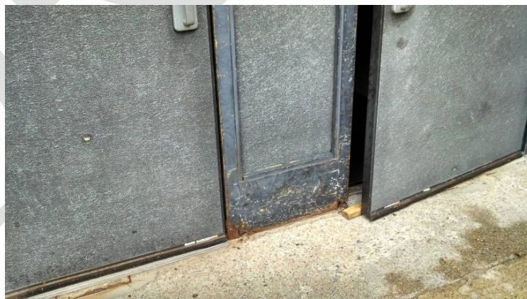
1956 Building original metal doors exhibiting rust
