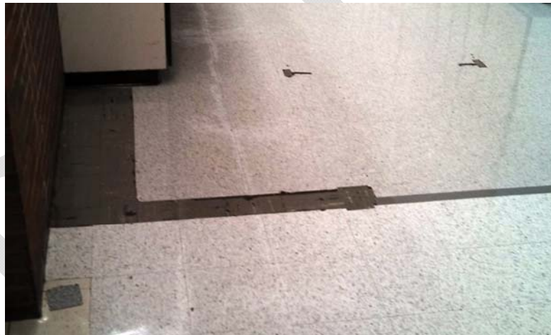
Patched or mismatched tile infill
