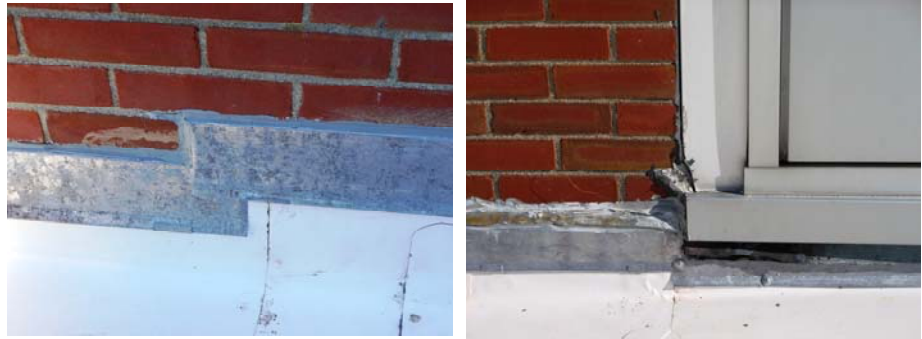
New sealant added as a temporary solution blocks weeps creating water issues within wall
