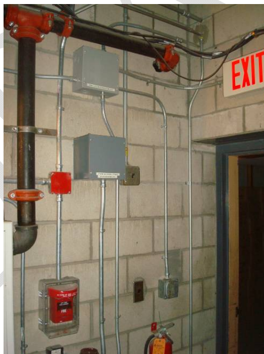
Stage Entrance and Bypass Relays
