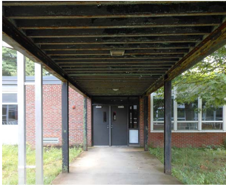
Northern courtyard breezeways with rusted structure
