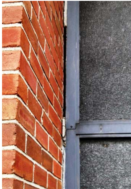
Exterior door systems showing portions of caulking completely missing
