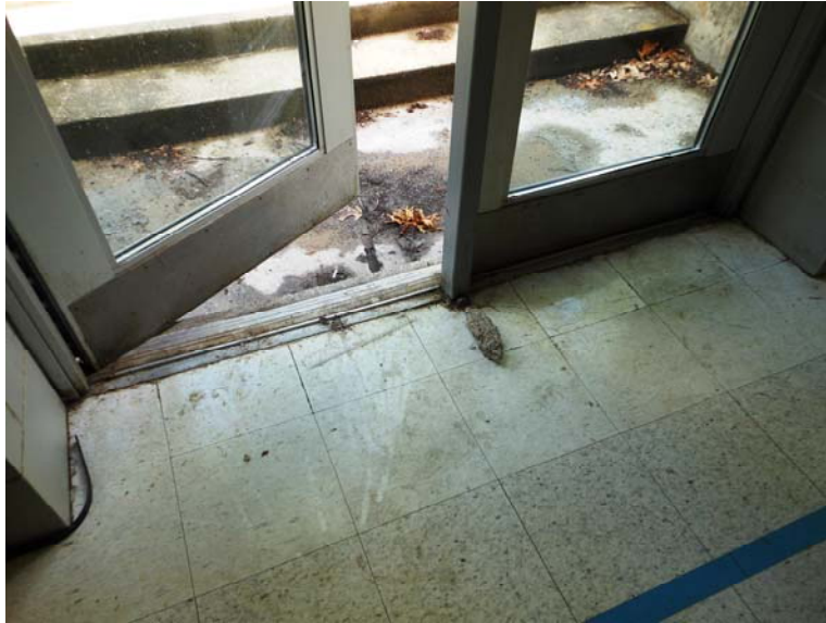
Northwest corridor water infiltration concern area
