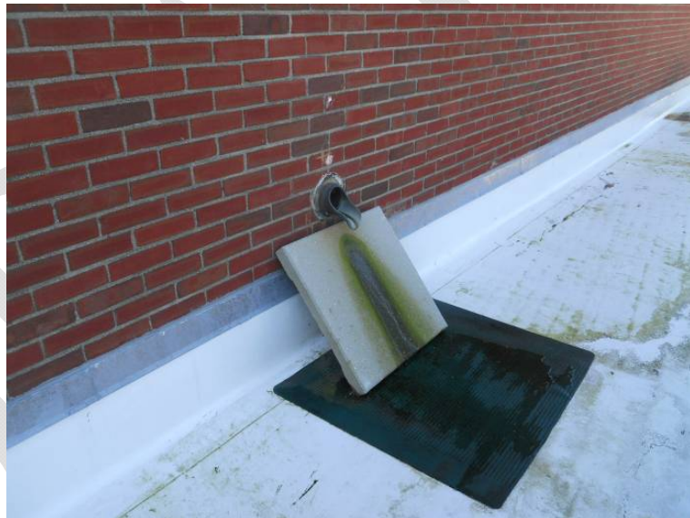
Roof overflow drain dripping onto make-shift splash pad
