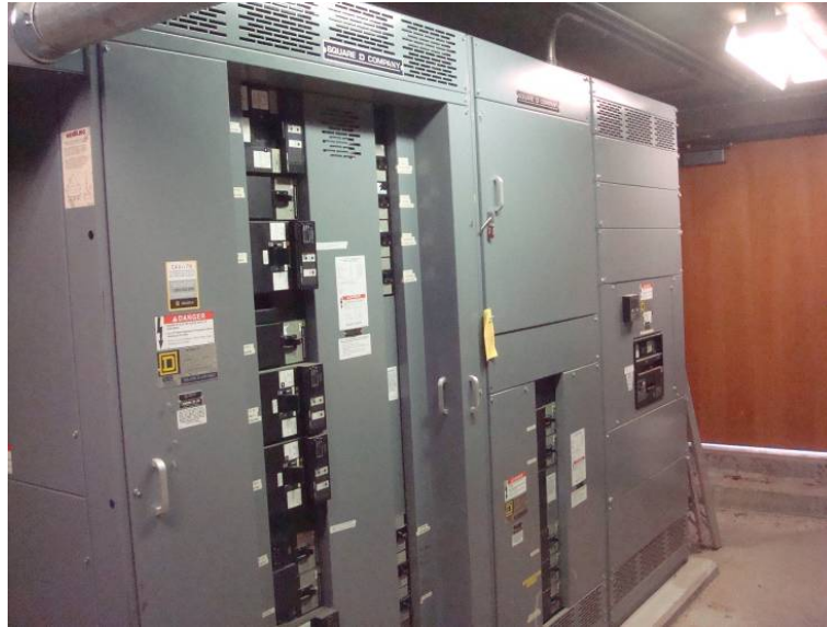
| Main Electrical Switchboard
