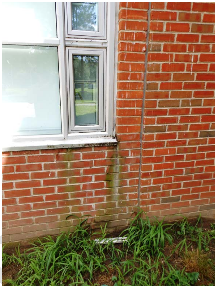
Moisture damage to wall because of storefront caulking and overlaps Efflorescence on the exterior wall and snap-on mullion removed and sitting on the ground
