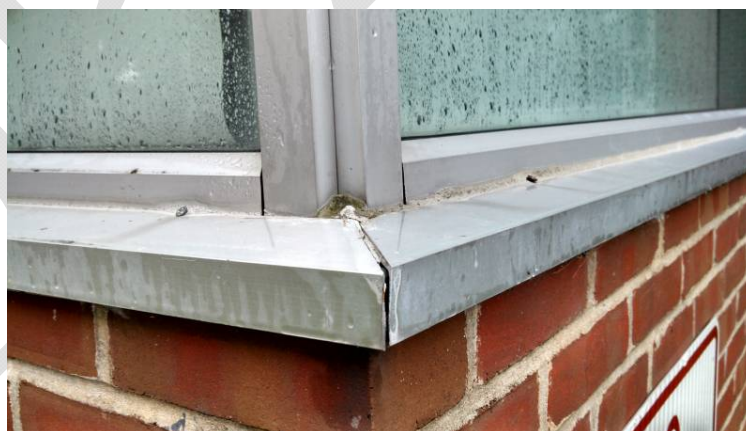
Exterior sill extrusion with missing caulk and rusty screws
