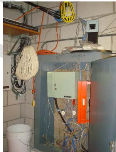
| Verizon Demarcation Point in Main Trunk Room
