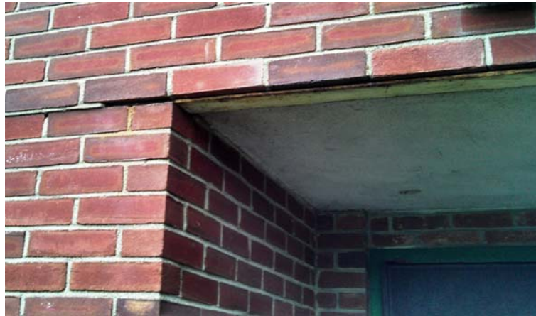
Rust jacking at the exposed steel lintel
