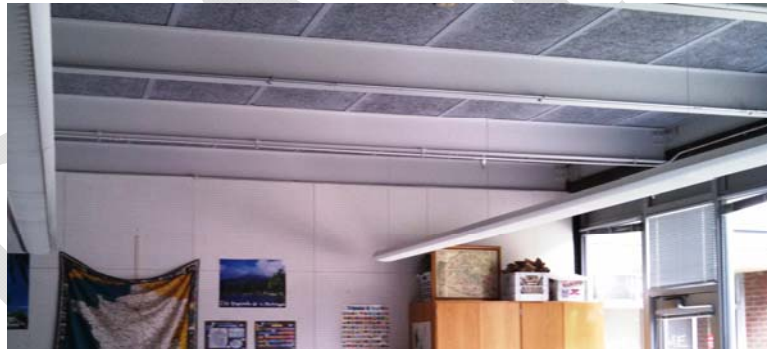
Typical classroom ceiling with exposed shredded fiber board
