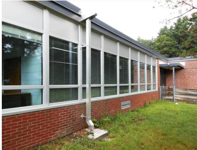
Typical scupper with stone splash pad
