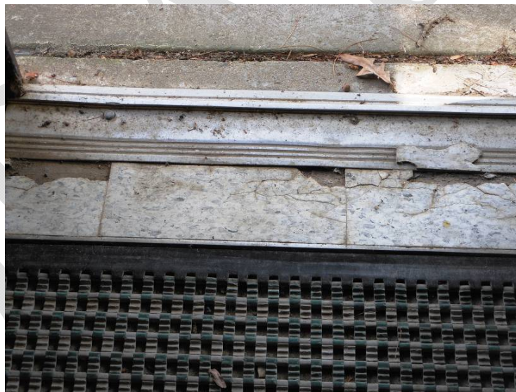
Exterior door showing damaged floor tiles and threshold
