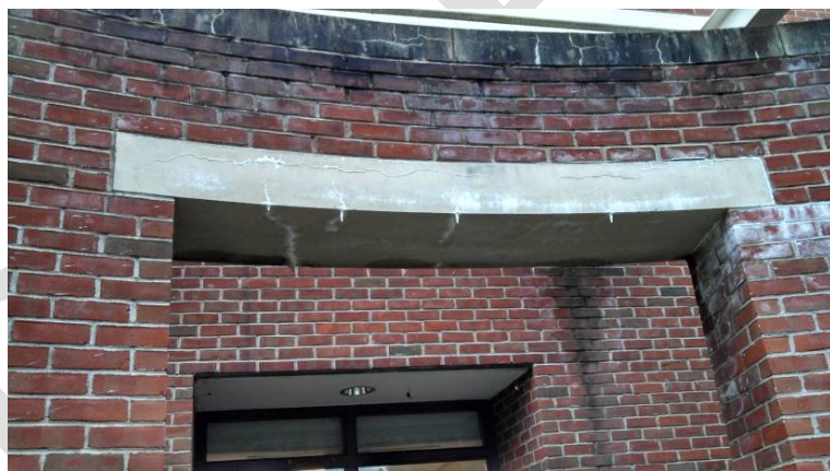
Efflorescence seen at building entry archway
