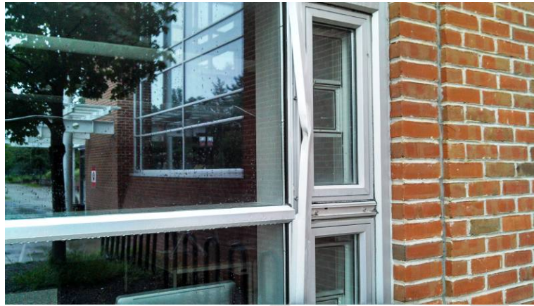
Damaged snap-on mullion cap
