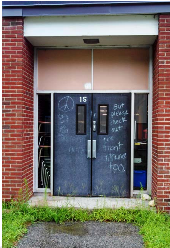
Typical exterior door showing step down, overgrowth, and damage
