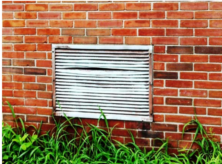
Bent blades on mechanical louvers
