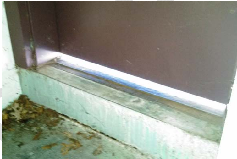
Gap at base of roof access door for water infiltration
