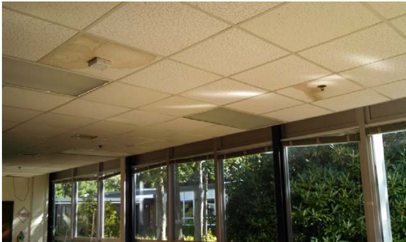
Damaged and mismatched ceiling panels
