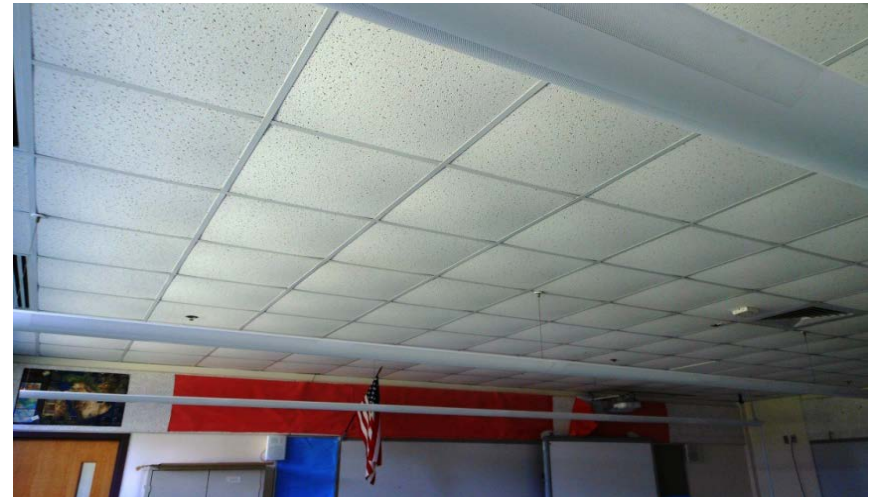
Bowing ceiling tile due to high level of humidity
